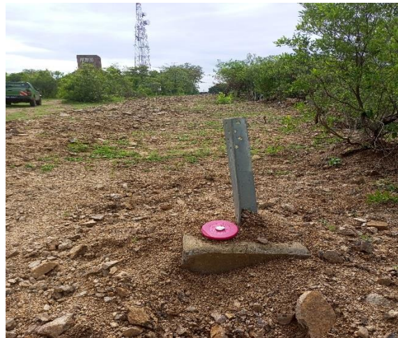
Tower 65, Stub twisted and deformed
