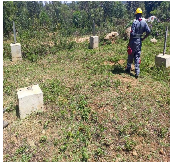
Tower 47, stub A deformed and cut
