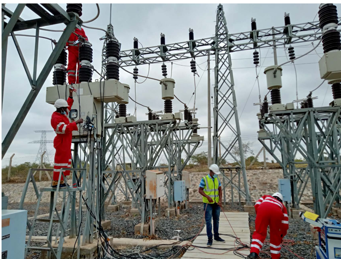
KETRACO O & M team servicing a circuit breaker at Kibos Substation
